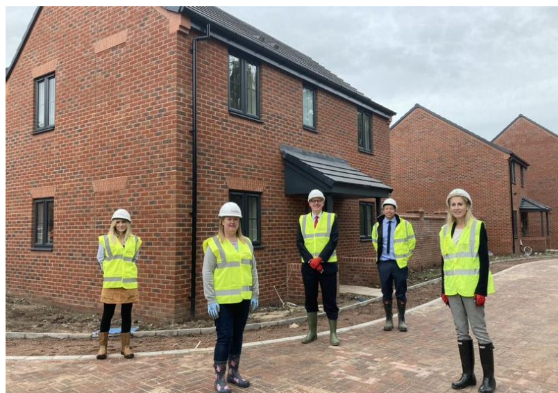
Homes under construction at Maple Fields, Dothill
